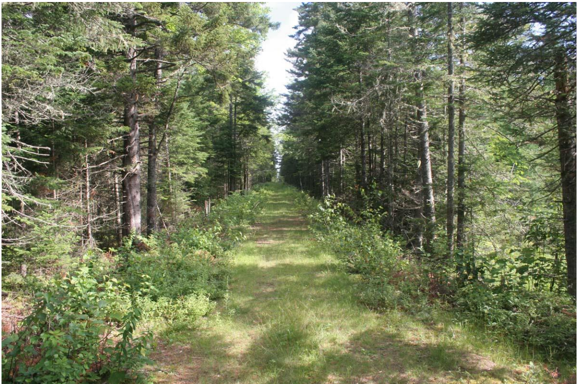
Photo # 8 description: Character of ROW 7500' south of Trudeau Rd. crossing, Bethlehem. 50' north of Beaver Brook bridge. Location of Beaver Brook overflow; consisting of two new 48" CMP culverts.
