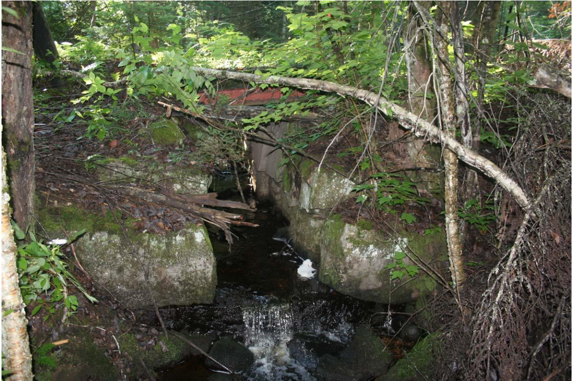
Photo # 3 description: B&M Bridge 222a, Bethlehem. 500' south of Trudeau Rd. crossing. Wood stringer on split fieldstone abutments, ~ 3' span. nd.
